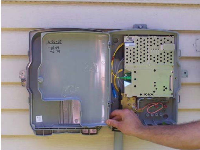
RUC's Fiber-to-the-Home Network Interface Device (NID)
